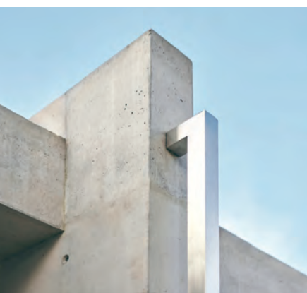
ABOVE: Downpipe detail.
