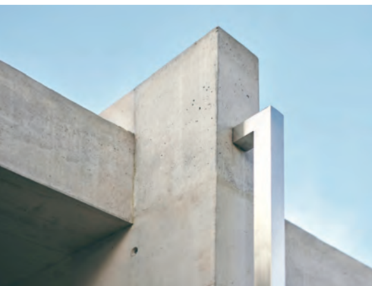
ABOVE: Downpipe detail.
