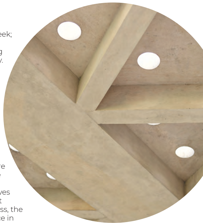
ABOVE: The coffered soffit.
