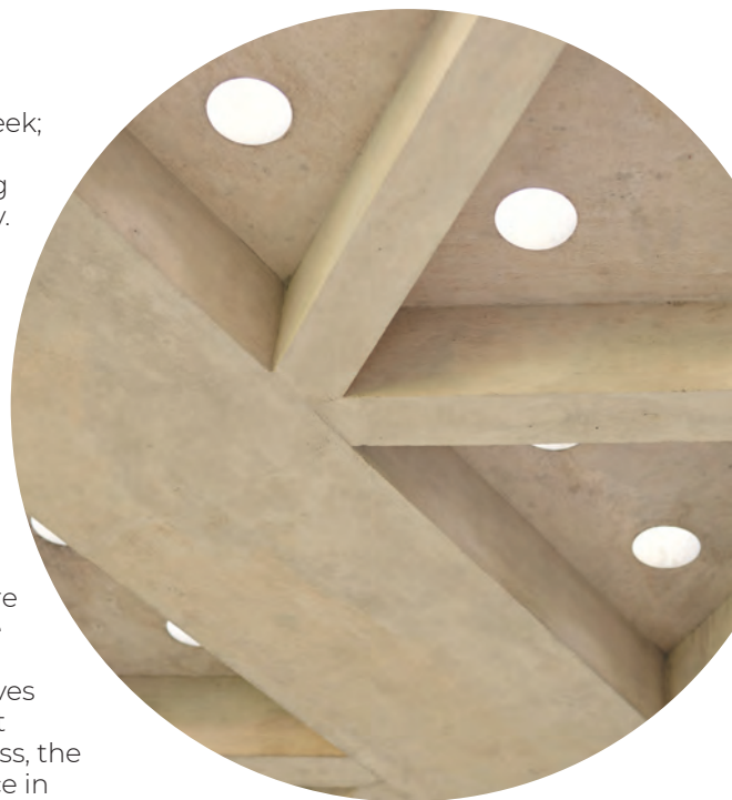
ABOVE: The coffered soffit.
